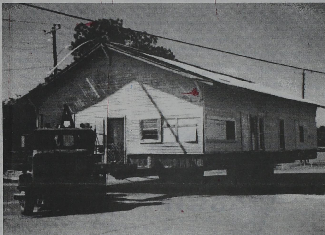
ON THE MOVE — The house of Denver Rainey that was located across the street from Maxfield Elementary is being relocated on Denver's farm outside of Gorman.
