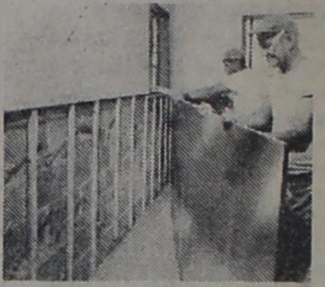
3. VAPOR BARRIERS — Beat the heat and the cold as well, with Foil-Back Gypsum Panels. The aluminum surface reflects heat rays, lowering indoor temperatures.
