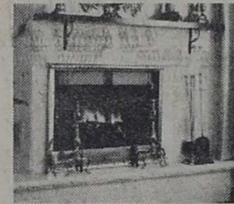
10. CIRCULATING FIREPLACE — This fireplace offers the advantages of heating and circulating warm air through individually controllable vent and ducts.
