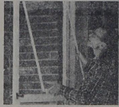
2. STORM DOORS & WINDOWS — Storm doors and windows can help reduce total heat loss by as much as 10%. Insulating glass and insulated doors help, too.
