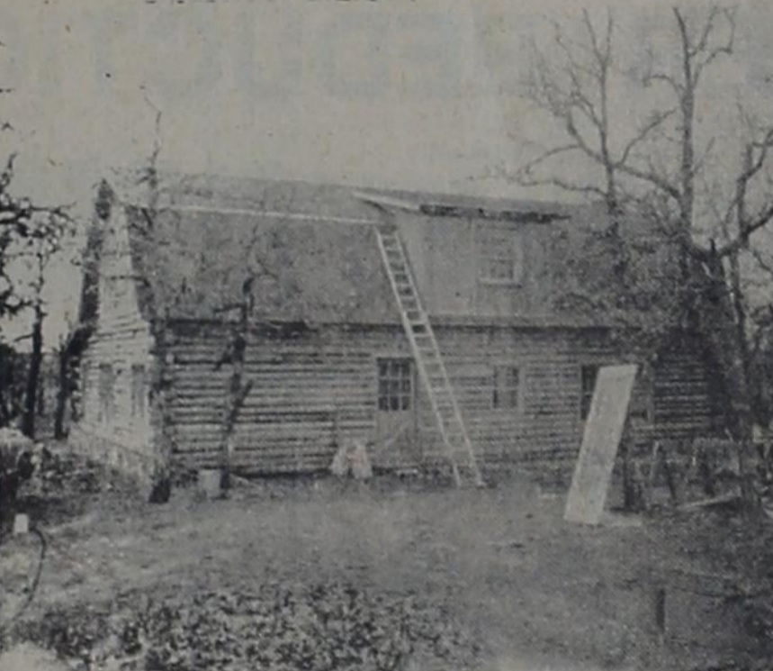
HARRISON'S HIDEAWAY — Pictured above is the new home of the Tommy Harrisons being built on the Duster Highway. Sorry we didn't catch Tommy on the ladder but he was on his way to work when the picture was taken.
