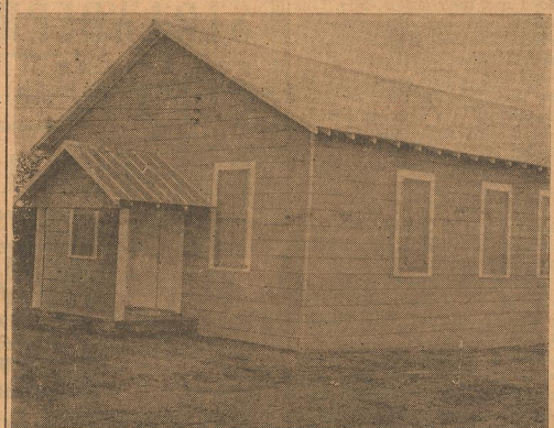
IMPROVEMENT AT KOKOMO COMMUNITY CENTER — Shown above is the Kokomo Community Center after the remodeling project was completed recently.
