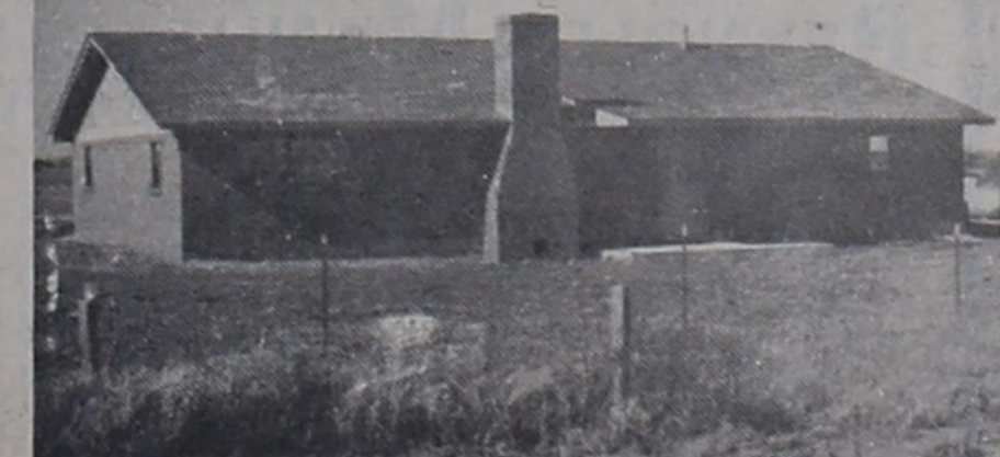
NEW HOME - Shown above is the new home of the Ronnie Weehunts in the Leon-Oliver Springs area. It is located on the Mears estate and is the completion stage.
