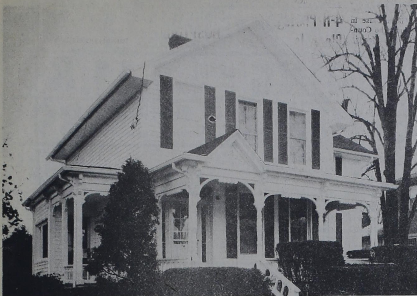
Older homes with beautiful architectural detailing can have easy exterior maintenance. Vinyl siding and accessory trim, such as that by Mastic Corporation shown here, have given this American clapboard home a fresh, low-maintenance look without destroying its architectural beauty. The contractor on this re-siding was D&D Builders.
