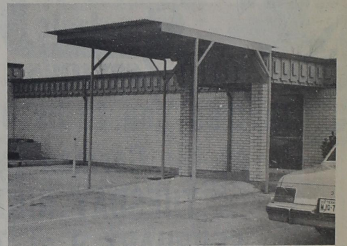
New Emergency Entrance covered shelter built by Auxiliary
