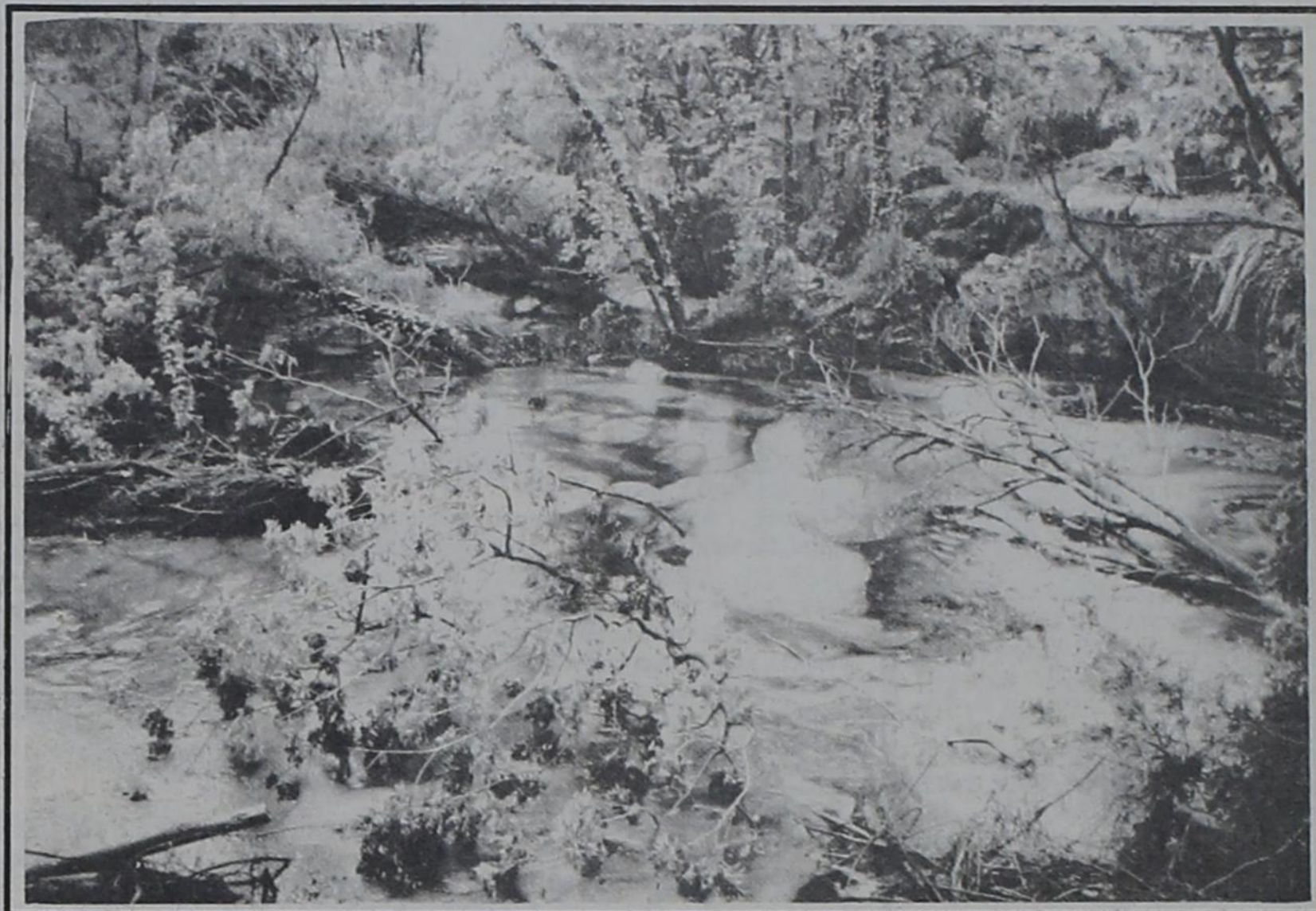
OIL SPILL RESIDUE -- Shown above (in center of photo) at Frank Gray Park is a huge glob of oil being swept away downstream by the rushing flood waters Thursday morning. The oil spill caused an overwhelming amount of damage to the park and downstream area.
