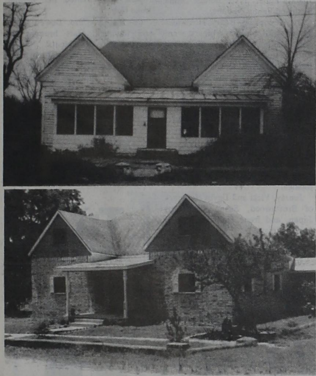
Shown above is the "before" picture of the Tommye Haile home on West Ross. The picture below it shows the new look of the beautiful home after the renovation project was completed. The construction work was done by T. J. Clark Construction of Gorman. Tommye and Erin are extremely proud of the "new look."
