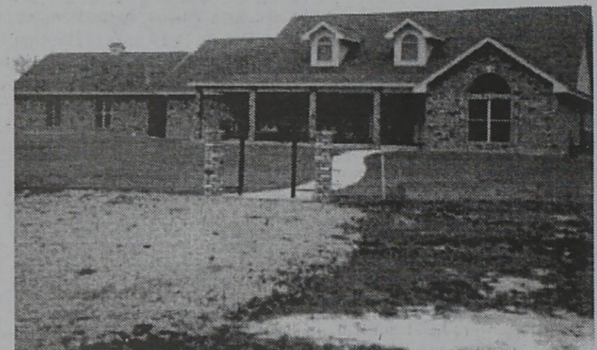
New Home For Jerry and Virginia Skaggs on Hwy. 6 West
