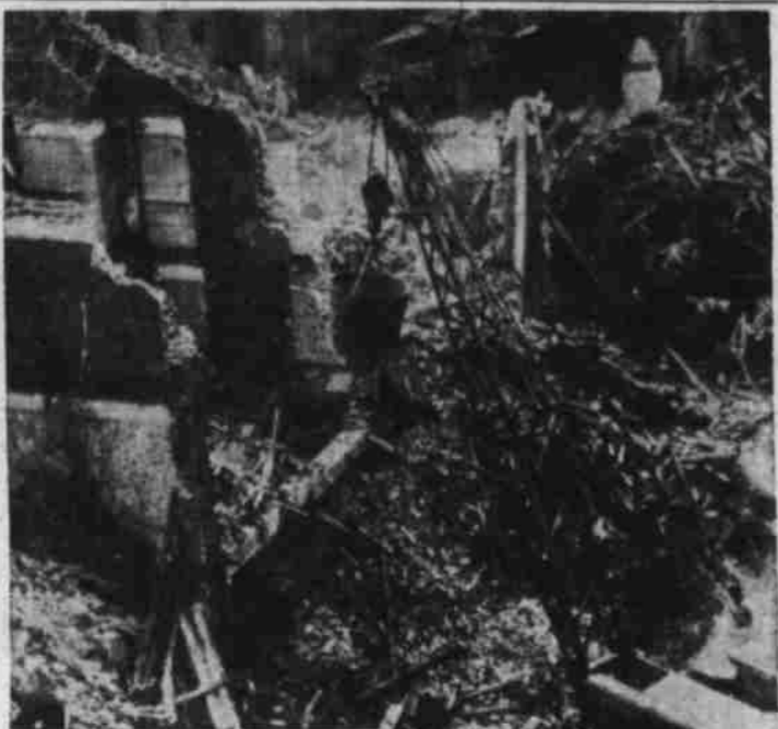
RESCUE WORKERS CLEAR WRECKAGE — Within a few minutes of the explosion of a German buzz bomb, work of rescue squads begins. Heavy equipment is put into use in search for possible victims and clearing of debris. (AP Wirephoto.)
