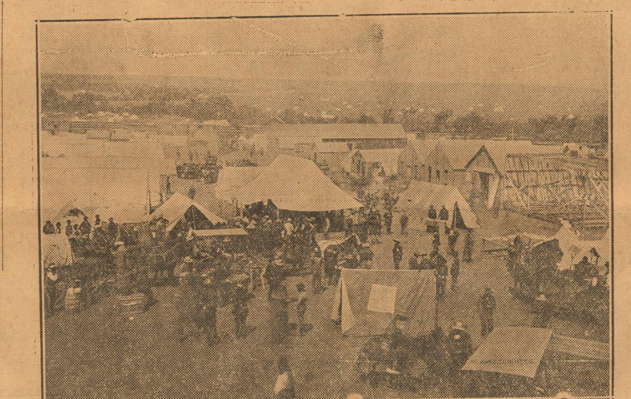
Guthrie on the fifth day, showing building construction.
