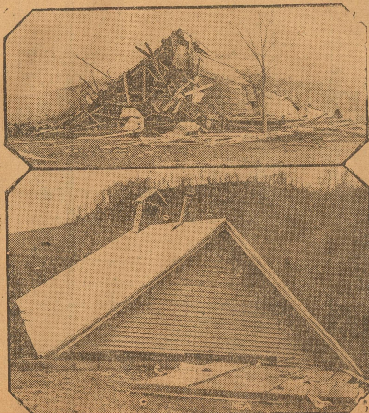
Wreckage of the Holmes Creek (Tenn.) schoolhouse, in which four children were killed in the recent tornado, is pictured in the lower photo. The wreckage at the top is that of Prosperity Missionary Baptist church. The storm through the state wrought damage of more than $500,000.
