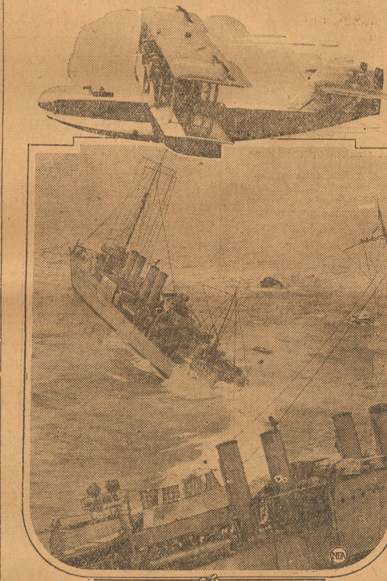
The wrecked hulks of seven U. S. destroyers, unpleasant reminders of the September night in 1923 when they were driven on the jagged rocks of Point Honda, Calif., carrying 23 men to their death, soon are to be blown to bits by a squadron of navy seaplanes from San Diego. Above is one of the bombers, and two of the wrecked destroyers as they appear today.
