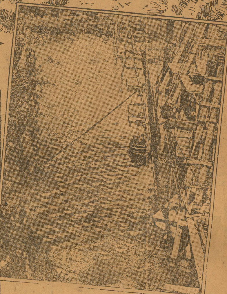
On false work and float the pipe line was carried before being dropped to the bed of the Sacramento River.
