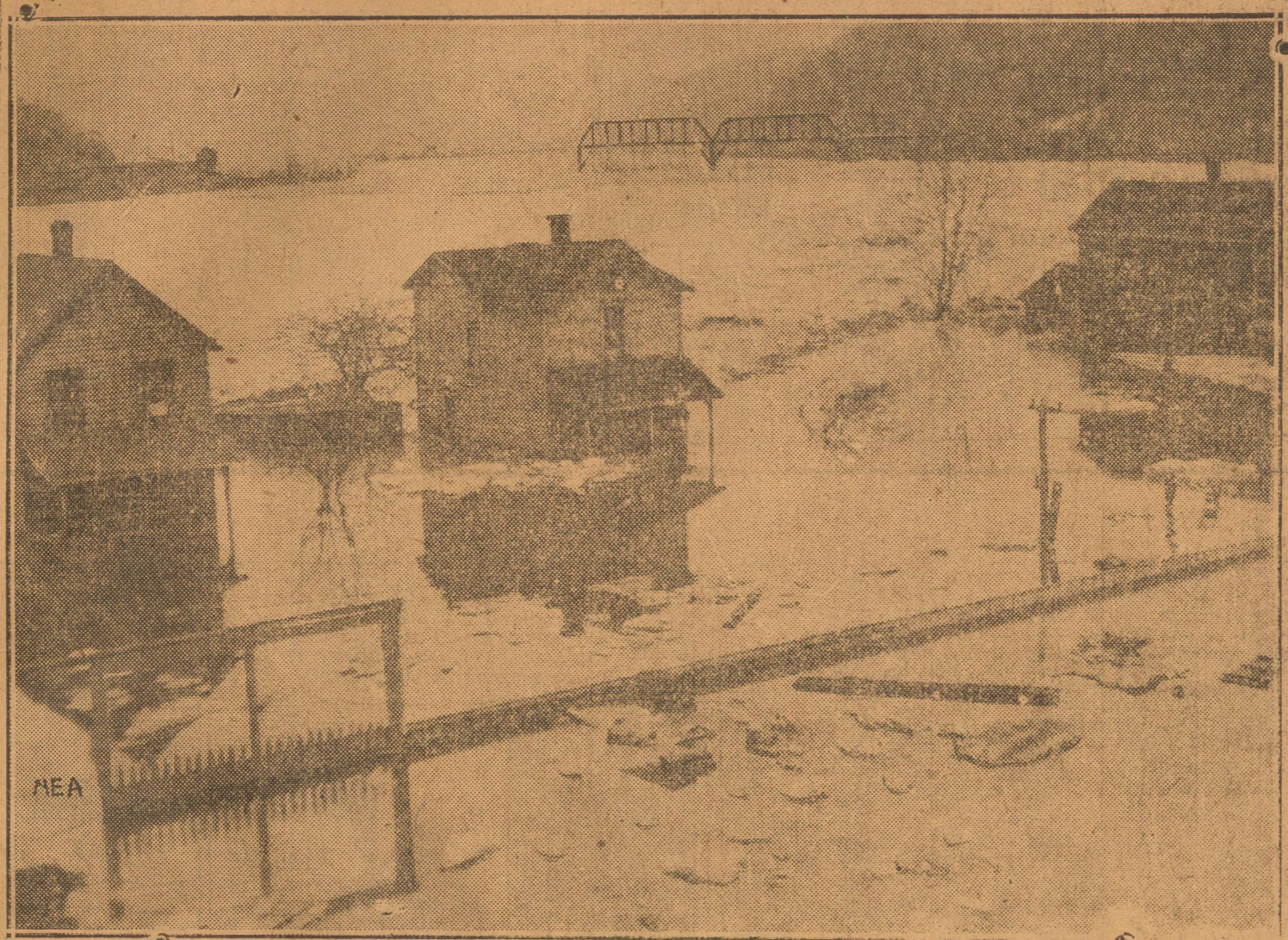
Here is how Elk street, Franklin, Pa., looked after ice jams in the Allegheny River had sent the flooded water over the banks. Photo shows the wrecked Big Rock bridge in the background, and gives an idea of how the water inundated the lower floors of dwellings in Franklin.
