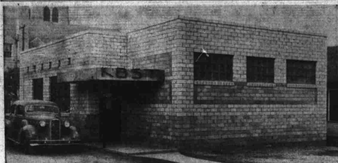
Modernistic Tile, Simple Lines—This construction, along with glass-brick windows, makes KBST's new studio building at 702 Johnson street an attractive and impressive building. Within, the building has everything one would expect in a strictly modern building. (Photo by Kelsey).
