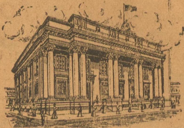
Main at Murphy Street
