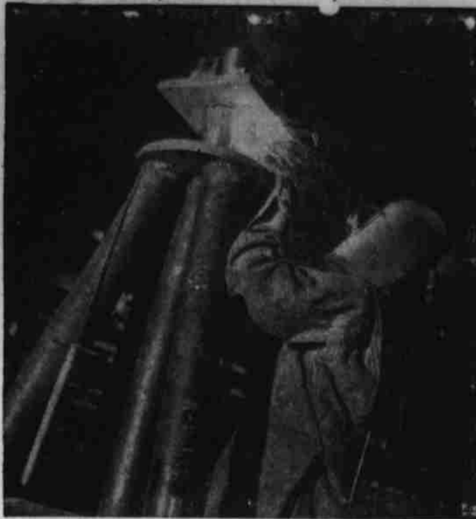
PLANE WELDER — Ray (Arky) Goodwin, 34-year-old welder, performs one of the delicate operations necessary to assembling a plane in Douglas' new Chicago plant. Welding is required to keep parts from shifting.
