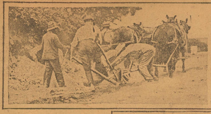
Plowing To Make a Road
