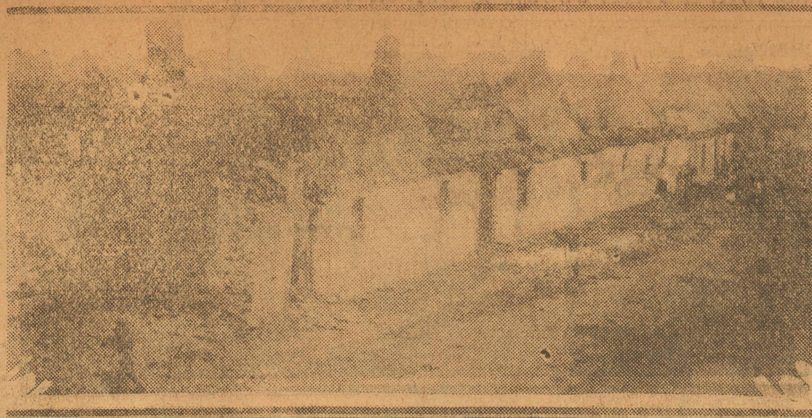
One row of wrecked homes.
