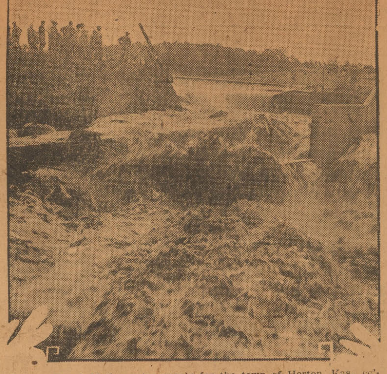
The dam that held the water supply for the town of Horton, Kas., collapsed after a series of heavy rains and every able-bodied citizen worked for hours to prevent the flooding of the town and destruction of crops. The lake that was released by the dam's collapse was two miles long, half a mile wide and 35 feet deep.
