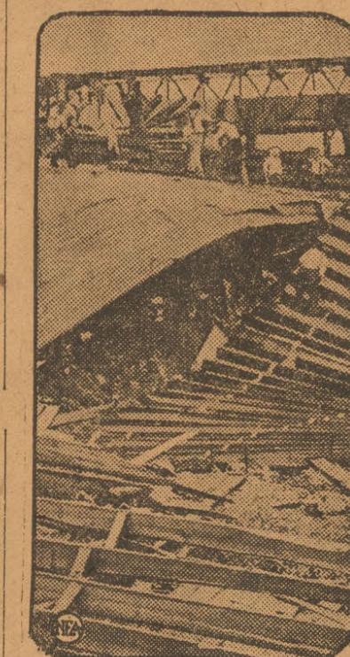
A baby cyclone swept down on Cincinnati and flattened out a good share of the buildings in the Union Stockyards with thousands of dollars' damage. This shows a small segment of the devastated area.
