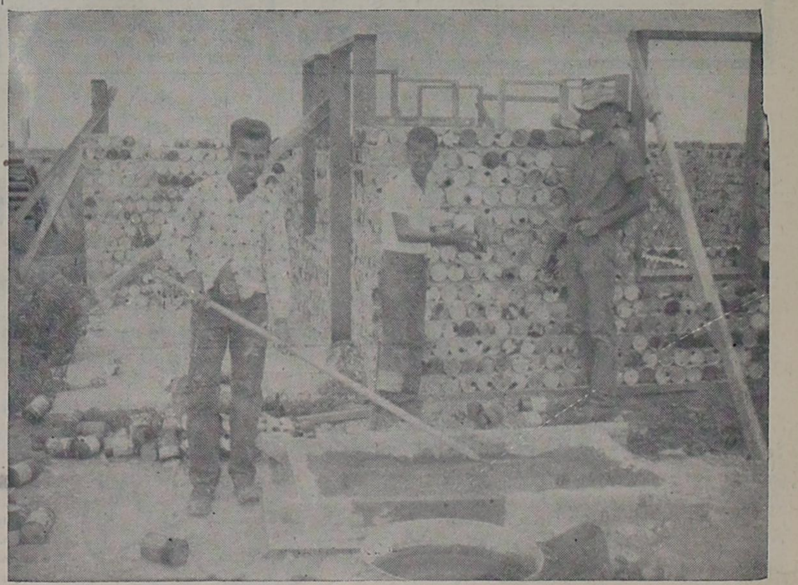
TIN CAN HOUSE—These three young men pause a minute as a photographer finds them hard at work, building a tin can house. Pictured, left to right are Billy, Johnny, and D. E., all sons of D. E. Hammit Sr., of Texico. The walls of the 25'x25' structure are all being constructed with oil cans from the Farwell dump ground.
