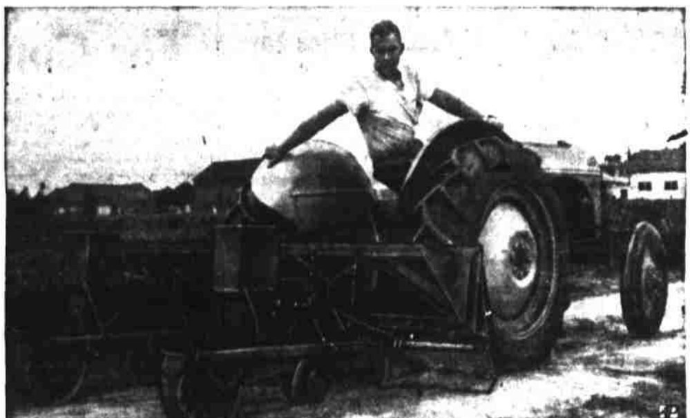
HIGH SPEED PLANTER —J. G. Futral, associate agronomist at Georgia Experiment station, operates the planter developed by him and Associate Professor R. L. Allen, of Georgia Tech, which will enable farmers to increase their planting speed from three to 15 miles an hour.
