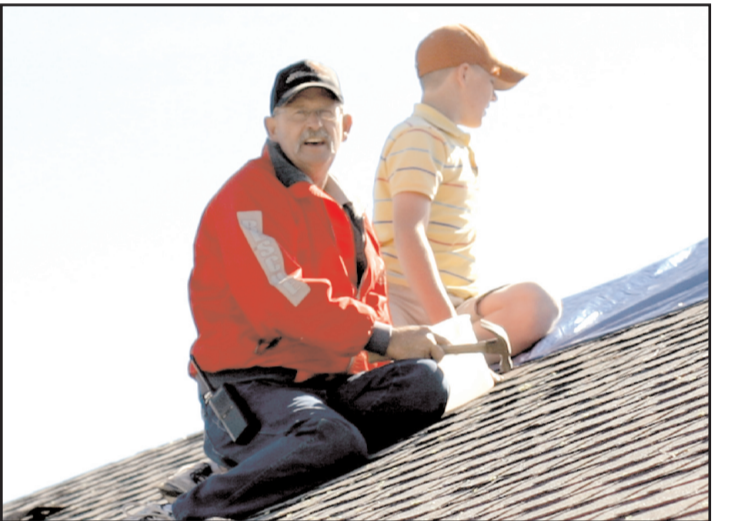
Jessie Stone and his son patch a hole in the roof.
