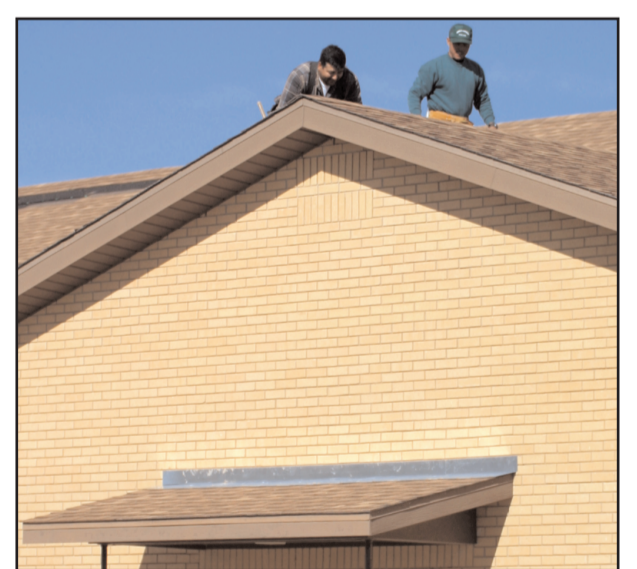
Workers repair the roof on St. Ann's Catholic Church.
