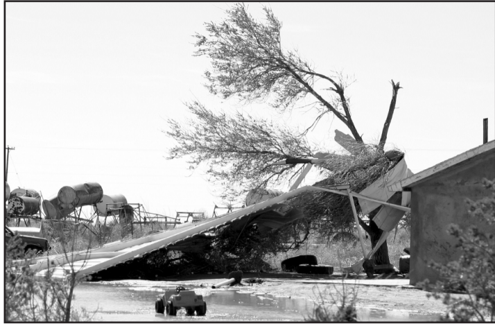
North of Bovina damage included this metal twisted by the storm.
