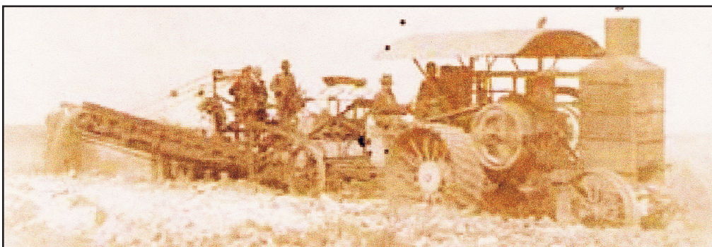
A 20 hp gas engine and grader. Written on the postcard is, "This will grade 1/2 mile average per day"
