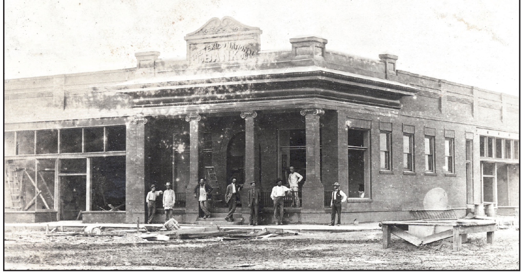
Workers construct the Texico National Bank. The building was established in 1908.
