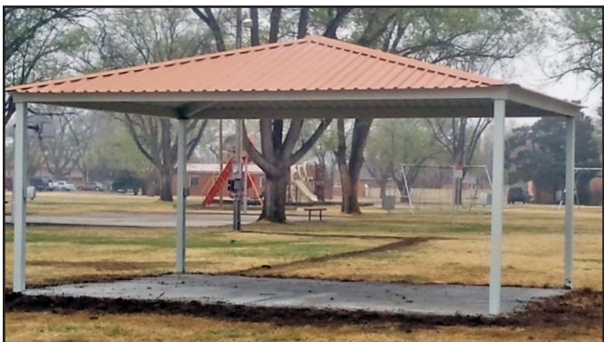
The new gazebo in city park has been completed with a concrete slab and electricity.
