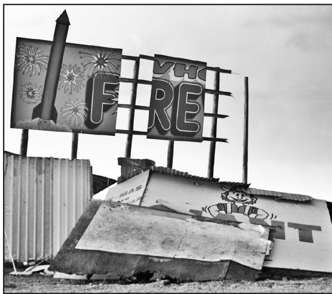
A fireworks stand is demolished
