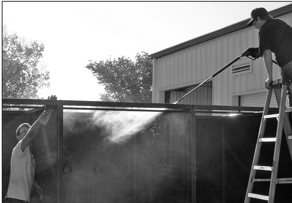
The boys work to scrub and remove contaminants from the steel prior to painting.
