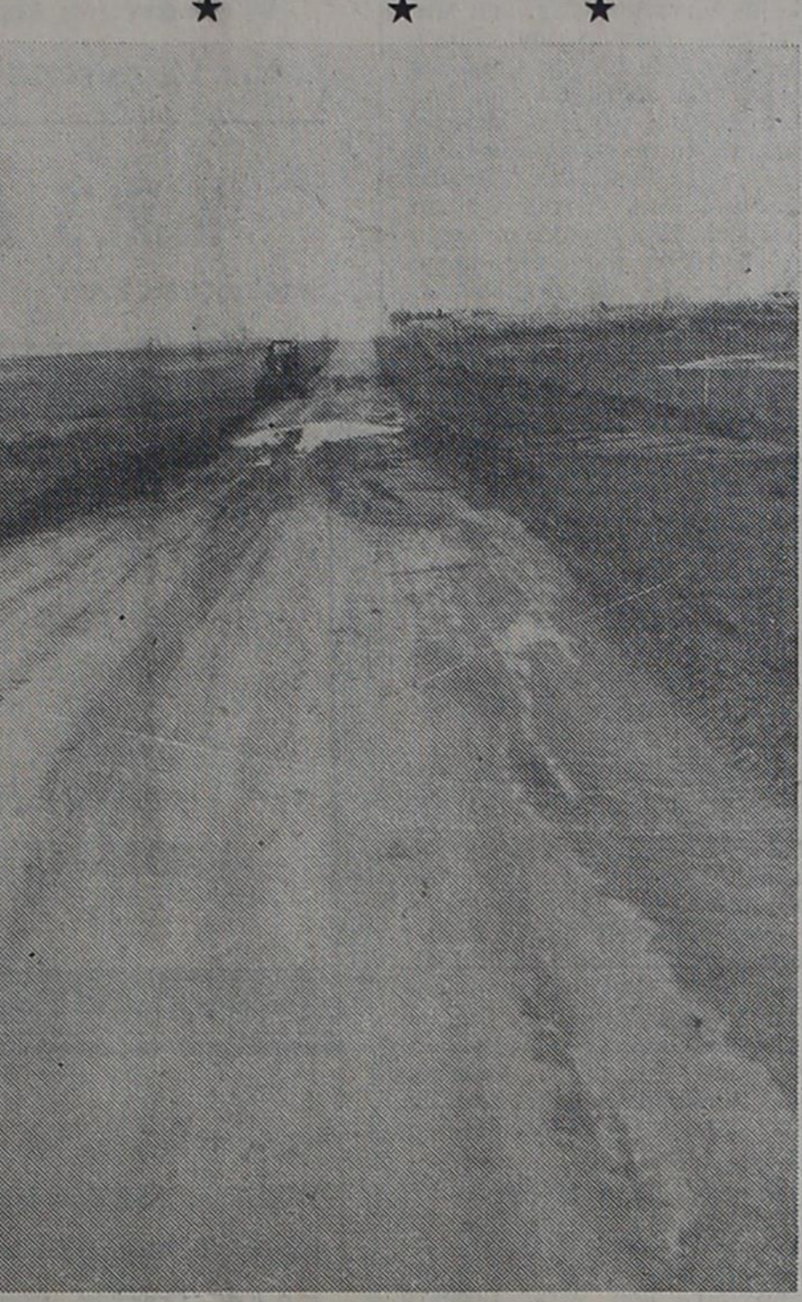
EROSION — An estimated five inches of rain Friday afternoon caused considerable soil washing south of Farwell. Here, a maintainer is scraping top soil from State Road just south of Farwell Feed Lots.
