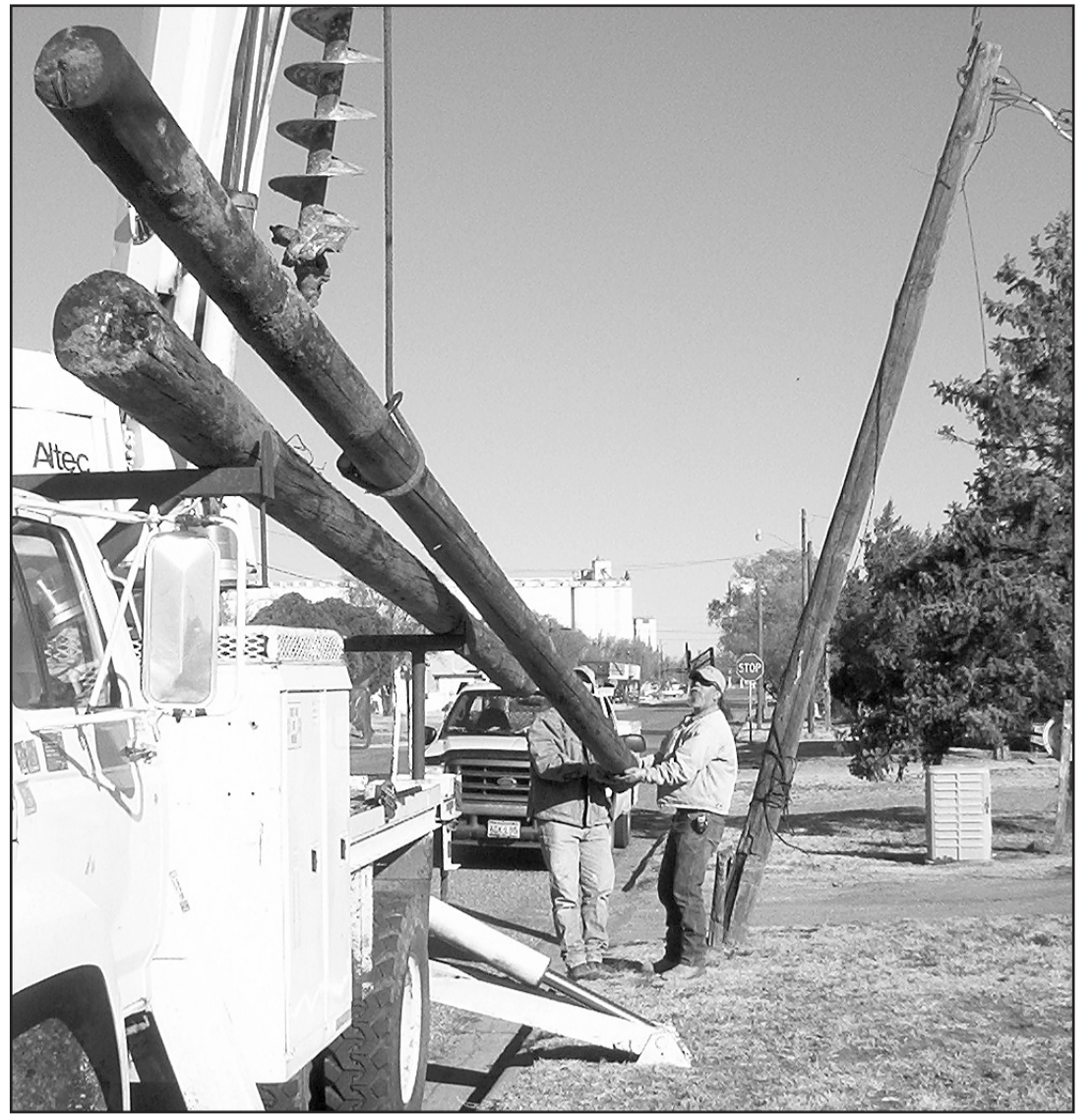
Campbell Electric workers placed a new cable TV pole in the 600 block of 4th Street in Bovina on March 30. A trash truck had clipped the old pole, causing the bend.
