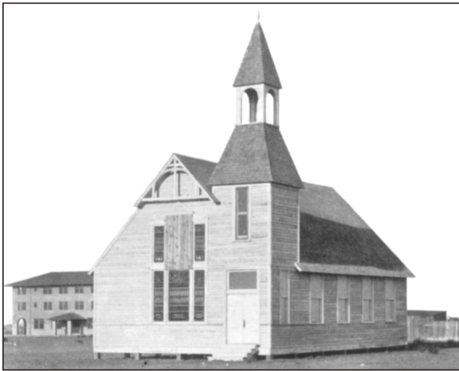
The Christian Church near 602 2nd St. The Farwell Inn is in the background.
