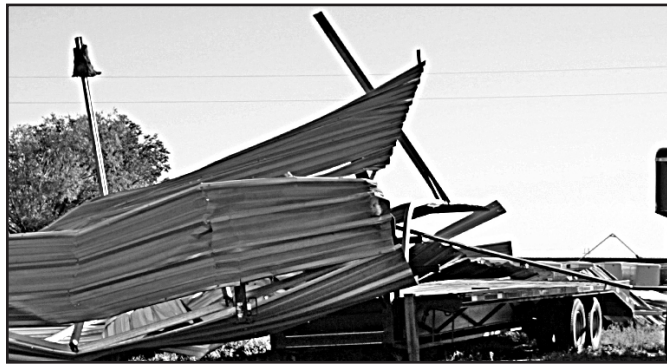
This post was ripped from the ground and the concrete footer was put on top of an undamaged shelter.
