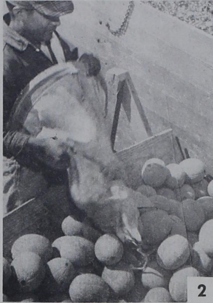
. . . and load them into waiting trucks.
