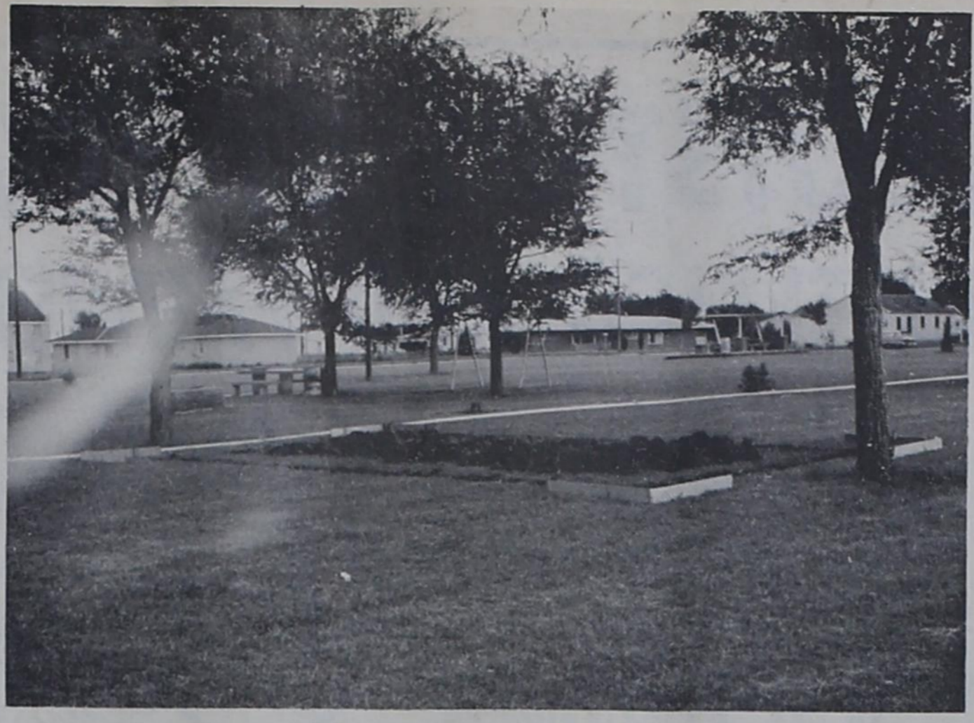
ONE OF THE NEW PICNIC SHELTER SITES . . . Shown is one of the sites of the four new picnic shelters now under construction in the Farwell City Park. Plans are for these to be completed within 30-45 days. These will bring the total of covered tables to five.
