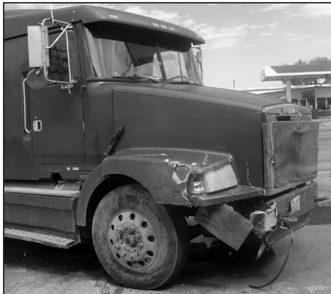
A two vehicle accident caused some damage to the Charles Oil & Gas building.
