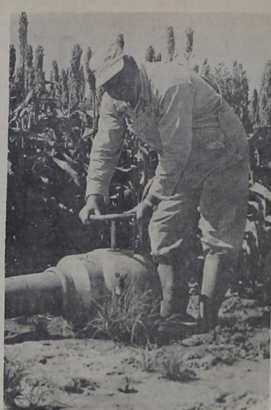
CONTROLLED IRRIGATION is made possible by an extensive system of underground pipe. Here Mabry opens a valve to release water to his thirsty grain sorghum.
