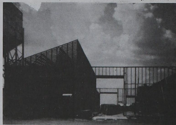
Terra's new fertilizer building.
