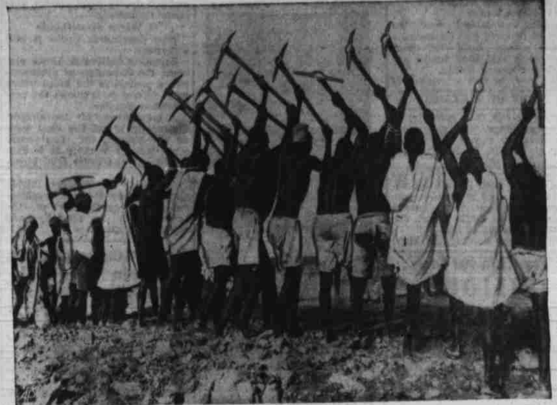
RHYTHMIC BUILDERS —Singing a Nile river boat song, natives of Nigeria, Africa, swing their picks in rhythm as they build an air base for the U. S. Army Air Forces.
