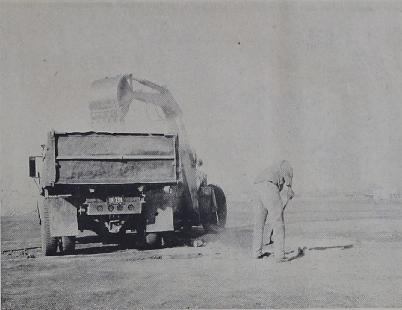
A backhoe dumps dirt into a waiting truck as workmen dig holes over which machinery and buildings will rest at the Tide Products, Inc., site on Highway 60. A large asphalt slab was run over the area 10 days ago.
