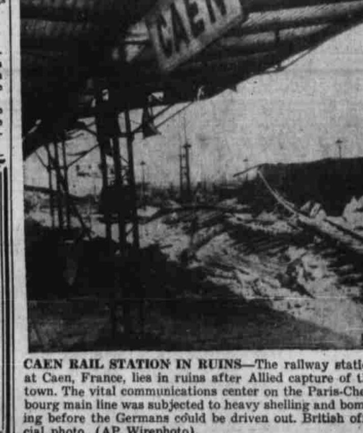
CAEN RAIL STATION IN RUINS —The railway station at Caen, France, lies in ruins after Allied capture of the town. The vital communications center on the Paris-Cherbourg main line was subjected to heavy shelling and bombing before the Germans could be driven out. British official photo. (AP Wirephoto).
