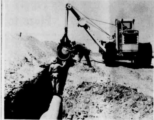
AFTER DELAY, WORK CONTINUES -- Workers had slowed the project Friday and Saturday. were moving on toward the sandhills with a 24- Shown here is a big side-boom rig which is used inch city pipeline this week after a legal hassle to lower the 30-foot lengths of pipe into the ditch.
