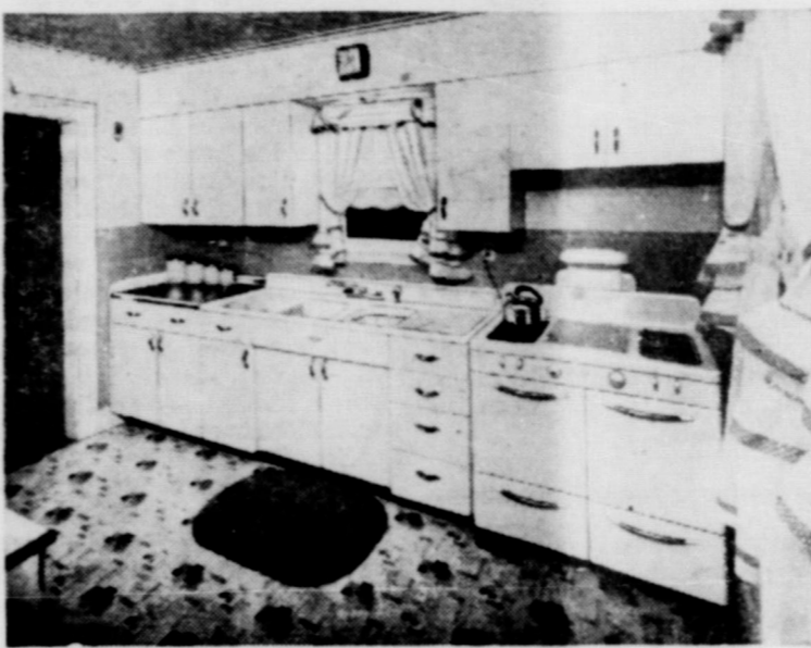
Symbolic of the transformation is the electric clock that replaces the old mantel timepiece. Alterations? Sure, but not expensive ones, because standard steel kitchen units were used and no structural changes were made. The window remains and the new cabinet sink was attached to the old plumbing. A soft light above the wall cabinets and the addition of wall tile are extra features. Note the large number of drawers and compartments in the double-bowl sink and base cabinets.
