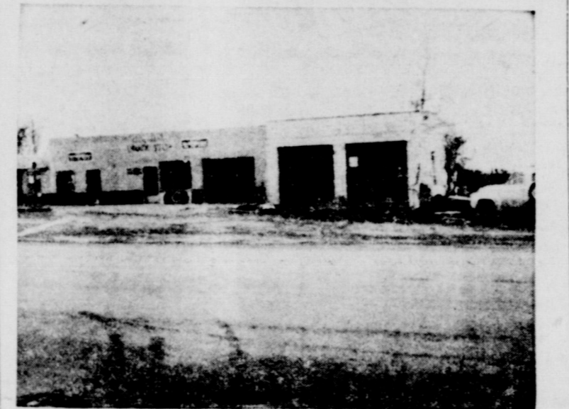
IMPROVEMENT: Another new improvement for Wheeler is this addition to Chapman's Service Station. Bill Chapman, owner of the station, has almost completed construction of a new wash and grease department to his service station. Chapman's place is located on the West edge of Wheeler.
