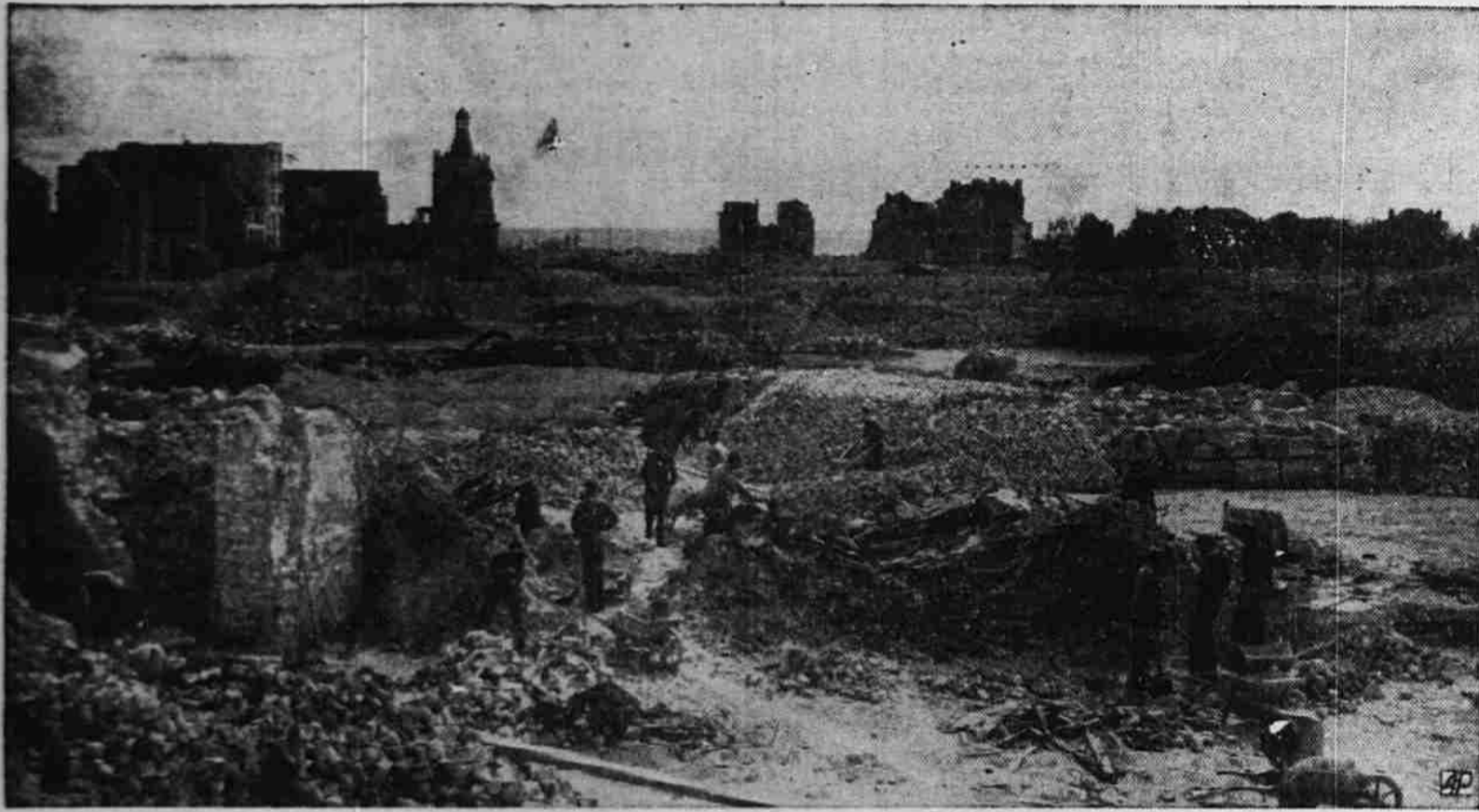
CLEARING DEBRIS OF SIEGE —At Le Havre, France's second port which underwent a long siege during the war, German prisoners clear away debris. The men sort out bricks and other building material for reconstruction.
