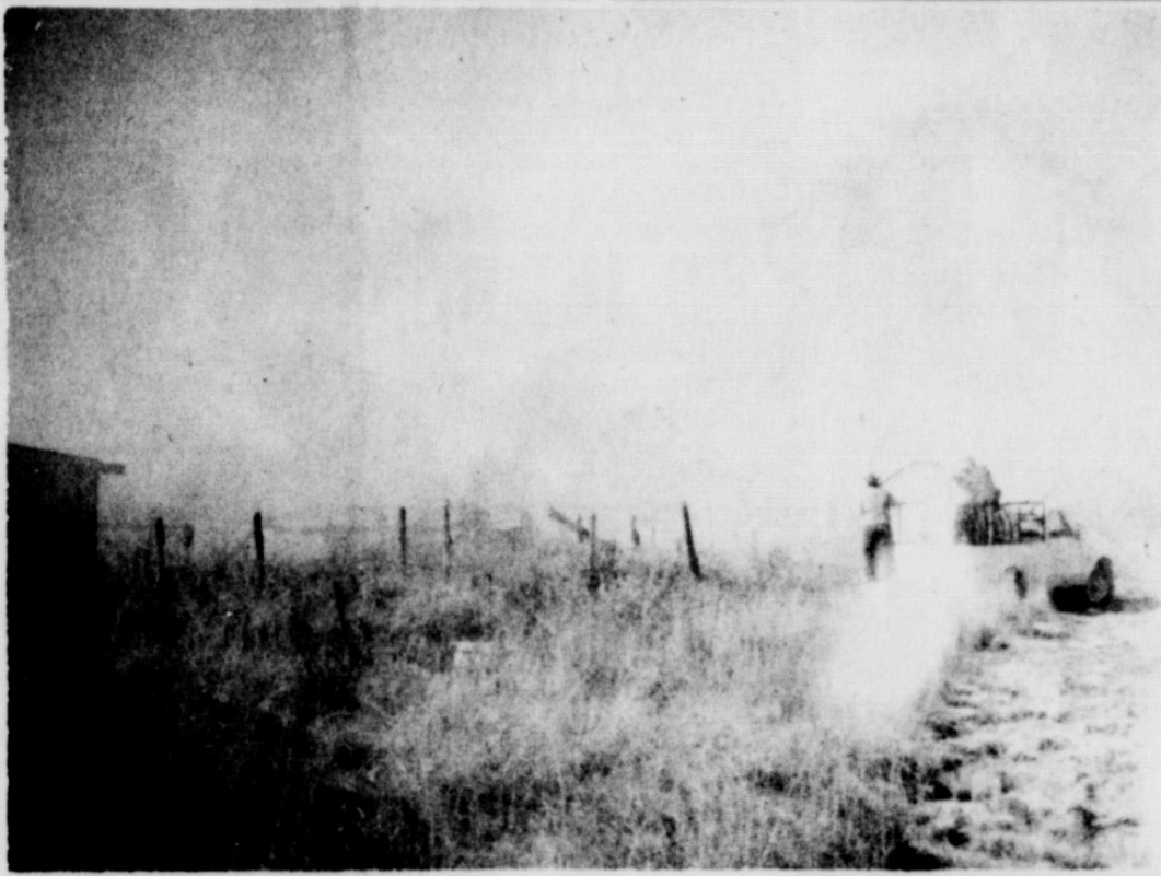
WORK BEGINS: Work has begun on the construction of a new Rodeo Arena for Wheeler. The new arena is being constructed on the south side of the present arena. It is hoped the work will be complete in time for the 16th annual rodeo in July. Wheeler Riding Club president, Gerald Johnson, stated the club will be happy to receive any donations—money, labor or material. The annual rodeo and barbecue promotes Wheeler in both business and public relations.
