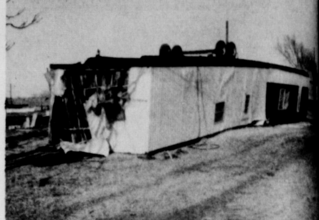
HIGH WINDS: A strong wind from the north Wednesday, March 31, toppled this trailer parked at the Sand and Sage Motel. The trailer, unoccupied, was totally demolished. The wind struck about 11:00 and flipped the trailer shortly after. Mrs. Joe Kelly received a sprained arm after her trailer was tipped by the wind. The Kelley's trailer is parked northwest of Wheeler.
