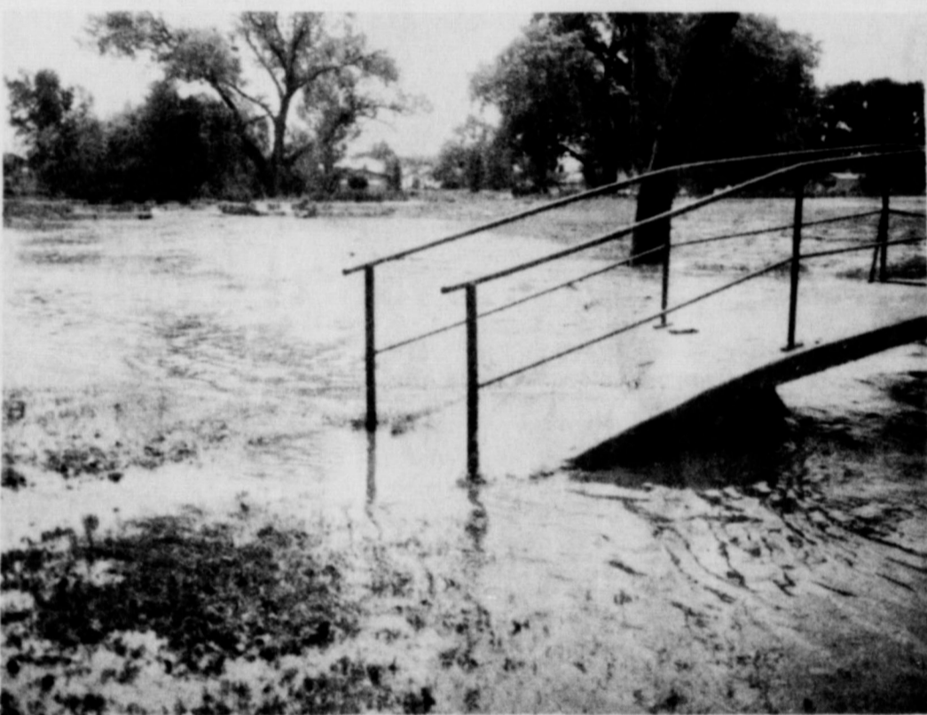
A LOT OF WATER: The foot bridge across the creek at the City Park was surrounded with water Thursday evening. The flood waters covered the bigger part of the park.
