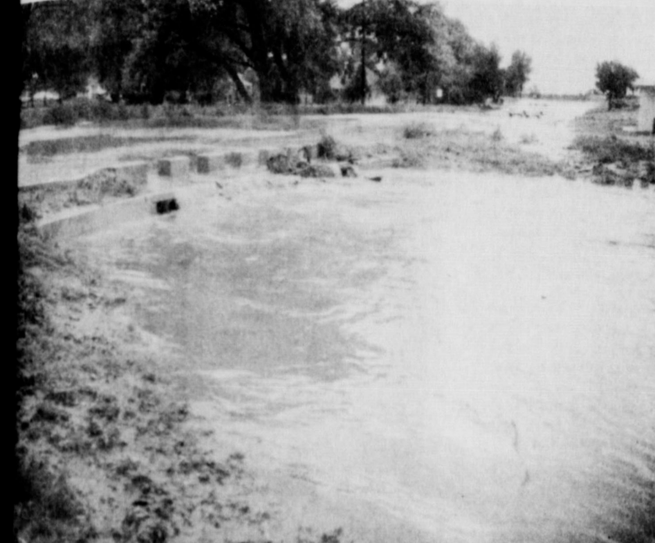
ON SEVENTH ST.: The bridge at the park was covered by the flood which resulted from the Thursday evening rain. The water was 6-7 feet deep a short time after the rain stopped. In the background is the 500 block of East Seventh which was heavily damaged by the water.
