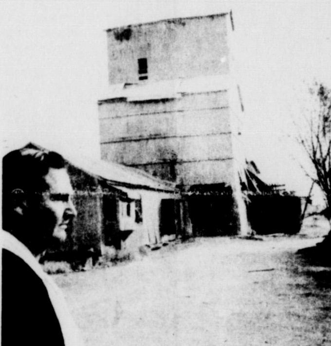
TALL BUT SHAKY - H. C. Johnson looks over the damaged remains of his Geronimo Elevator Co., elevator in Eads. The structure, located a block east of Main adjacent to the Missouri-Pacific tracks, was rocked by an explosion at 9 p.m., Thursday. Johnson's son, Steve, was severely burned in the mishap.
