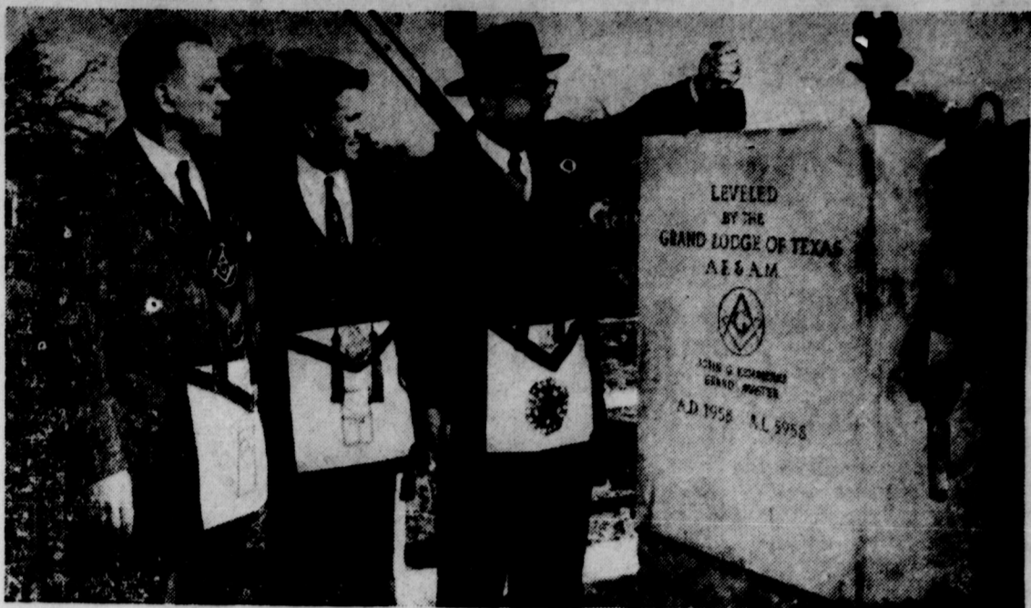
Among state officers of the Grand Lodge of Texas, A. F. & A. M., who participated in the levelling of the cornerstone for a new chapel building being erected on the campus of Masonic Home and School of Texas, located in Fort Worth, were: left to right, Randall E. Briscoe, deputy grand master, Houston; John T. Bean, grand senior warden, El Paso; John G. Kemmerer, grand master, Fort Worth. The cornerstone was leveled on November 29.
